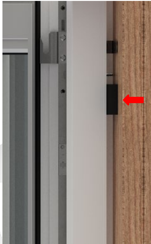
Figure 16: Jamb Shims
