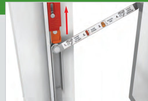
Step 2. Slide red cover up and hold.
